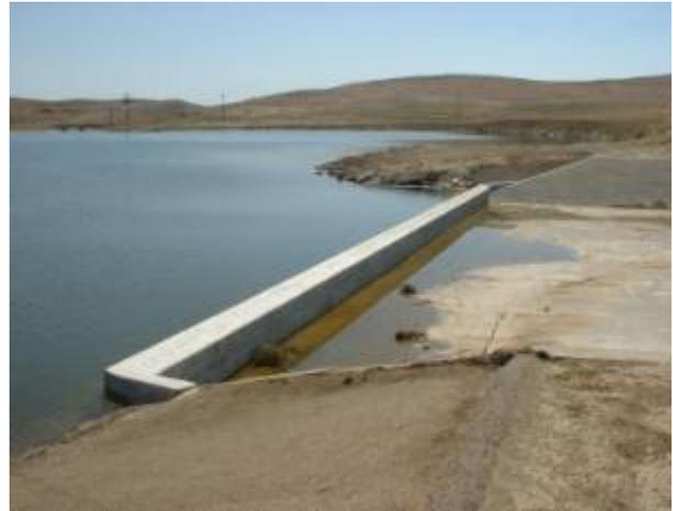
Figure 2. Increased height of bank at the reservoir inlet (top) and increased spillway height (bottom) in Berrenda Mesa Reservoir.
