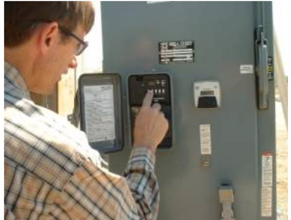
Figure 2. Clock timer used to automatically shut a groundwater well off before 12pm and turn it back on after 6pm every weekday during the peak season.
