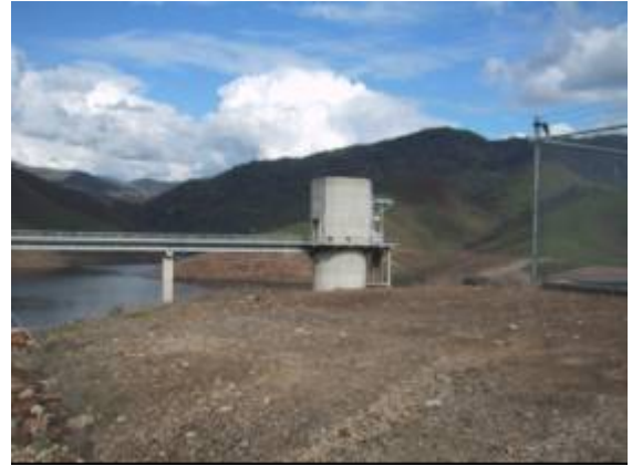
Figure 3. Inlet from Lake Kaweah to the turbine at Terminus Dam
