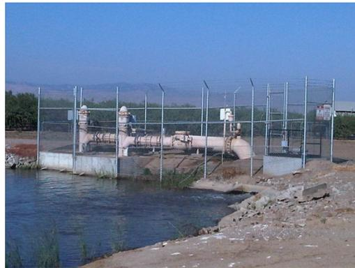
Figure 9. Pump station and valves to divert water from the reservoir into 3N or vice versa
