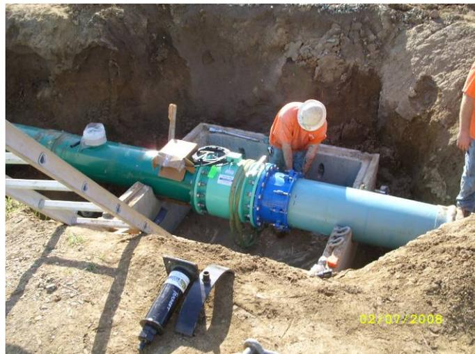
Figure 11. 1N pump station magnetic flow meter
