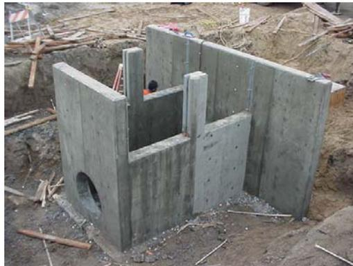
Figure 8. One flow control structure to the north of Fruit Avenue with weir length designed to pass high flows under system failure conditions.
