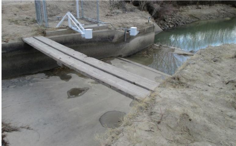
**Figure 1.** An existing Parshall flume that is frequently operated with downstream submergence in New Mexico. The initial installation omitted the downstream sensor. The downstream sensor was later added and the flow computation was adjusted to account for submergence when it occurs.
