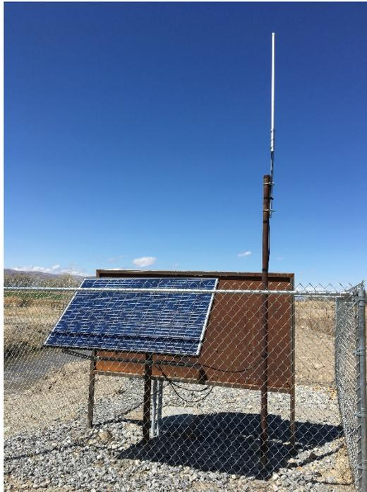
**Figure 5. Partial shading of a photovoltaic (PV) power system can be problematic and can sometimes be corrected with minor modifications. This PV panel in western Nevada is shaded most of the time by an adjacent fence structure.**
