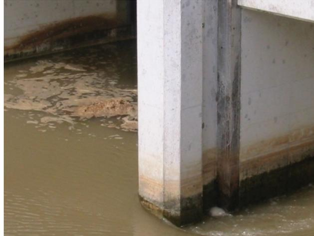
Figure 2. Noticeable head loss at the entrance of an upstream controlled gate structure
