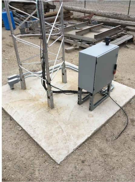
**Figure 6. The base of a 50-foot SCADA radio tower fitted with a single and undersized grounding conductor (seen in the lower right of the frame).**
