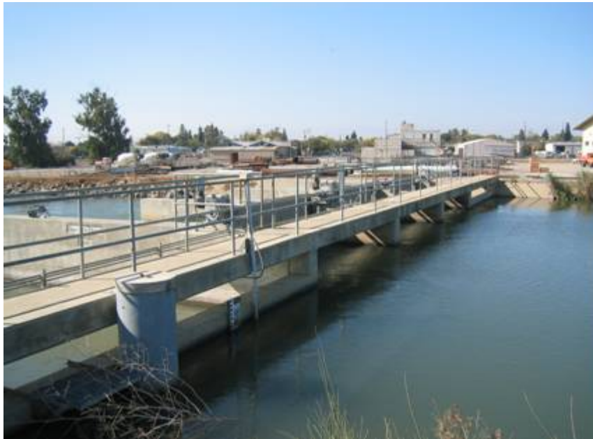
Figure 2. Willows Check on the GCID Main Canal
