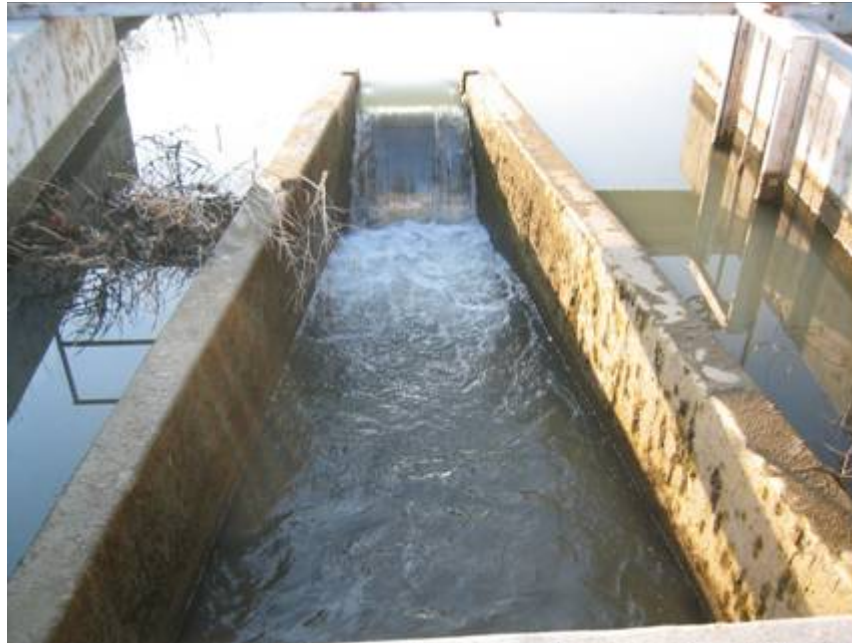
Figure 10. Demonstration long-crested weir in Lateral 59-1
