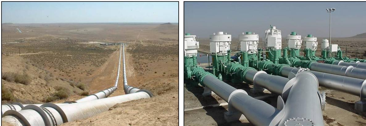
**Figure 1. Berrenda Mesa Water District's 9,900 HP (10 pumps total) pump station. With the CEC APLRP the district was able to curtail 4.67 MW of peak energy use, but in the past 2 years the increased demand from additional cropped acreage has led to more on-peak pumping.**
