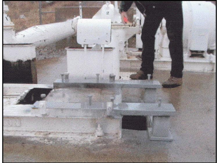
*Figure 3. Motor Stand Modifications at Roza I.D.
