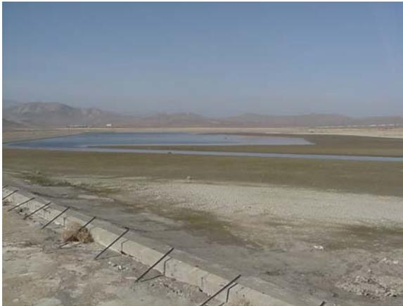
Modified buffer reservoir at Berrenda Mesa WD. Raising the spillway 15 inches increased the reservoir's holding capacity from 90 AF to 130 AF. An additional 40 AF will be obtained through excavation.
