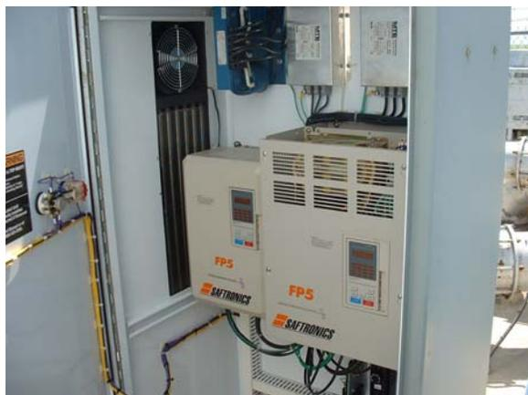
Two variable frequency drives at pump station C1. The station services two pipelines, with one VFD per pipeline.
